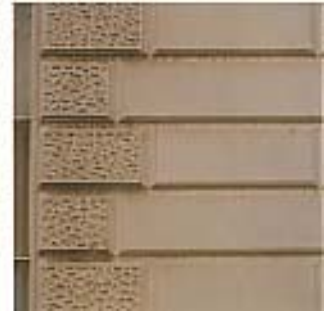
Chamfer bands with vermiculated quoins
