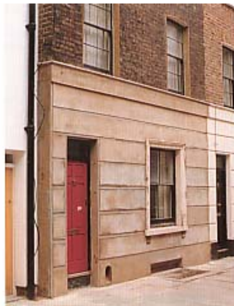
Middleton Buildings: Successfully detailed and finished reinstatement of band-rusticated stucco.
