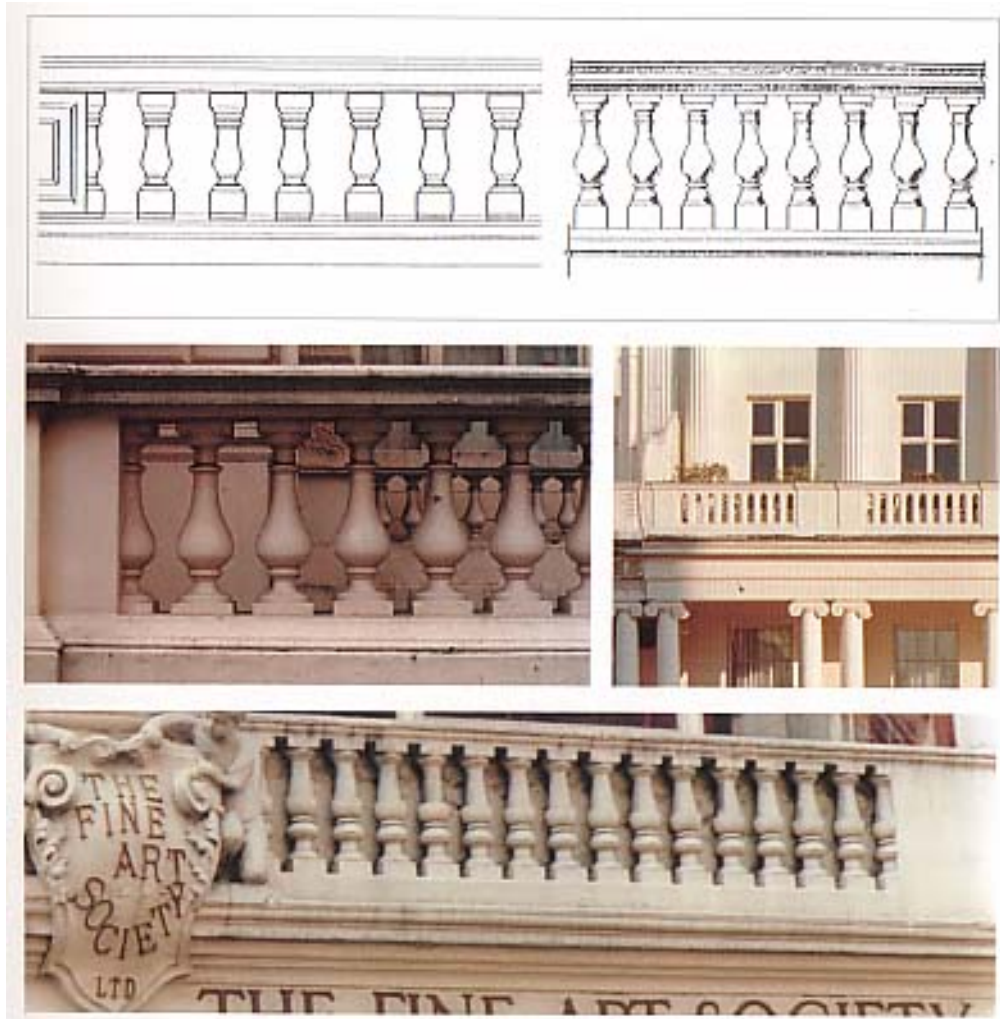
Examples of different types of balustrades on stucco buildings in Westminster.
