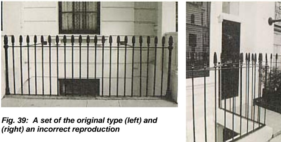
**Fig. 39: A set of the original type (left) and (right) an incorrect reproduction**
