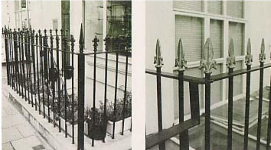
***Examples of mild steel replacement railings: Where consent is required for the installation of mild steel railings, the City Council will seek to secure that not only the heads and finials but also the size of the bars, their spacing and all structural details are made to correct authentic design. On listed buildings, the City Council may require the use of the original type of metal. The above two examples are not entirely successful.***
