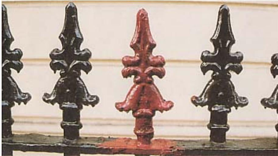
***Treatment and protection of rust affected connection point. Note the complete removal of old paint before the application of the protective primer.***
