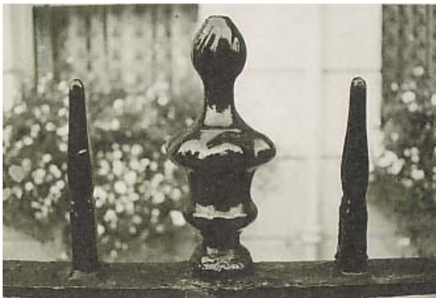
***An example of loss of detail caused by overpainting. Note the shrinkage of the paint at the base of the finial, usually caused by the application of thick layers of paint.***
