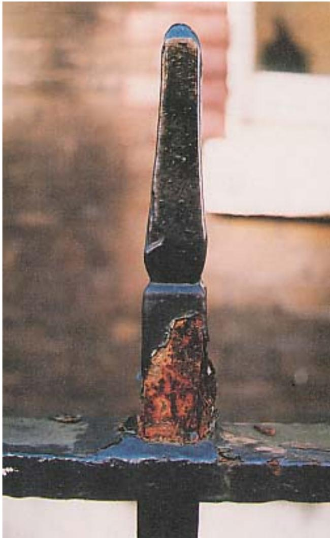
*Typical example of corrosion at points of contact of two different metals where different movement of two parts can cause water penetration.*
