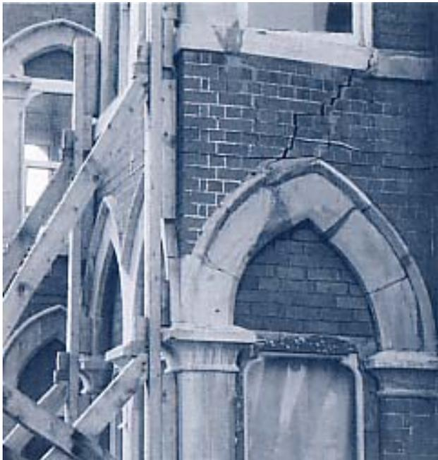
*Fig. 9: Structural failure of pointed arch and wall above, due to differential settlement between its two sides. This can often be the result of inappropriate strengthening of part of the foundations.*
