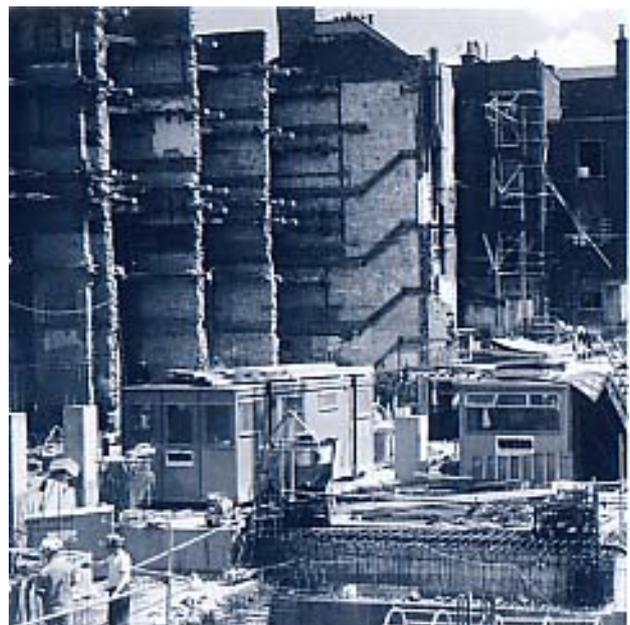
**Fig. 13: This example illustrates the right method to provide temporary support to a retained facade. This involves an appropriately calculated and constructed temporary structure, in this case consisting of steel members and frames.**
