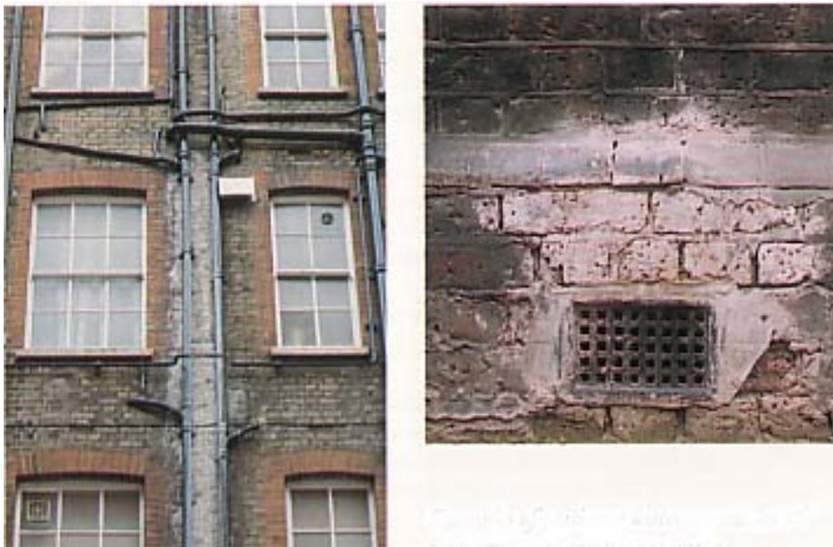
***Examples of persistent water saturation of brickwork and resulting staining.***
