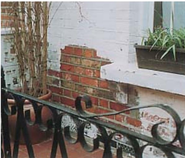
***Removal of paint from brick-facade (trial-sample) carried out with the poultice chemical method.***
