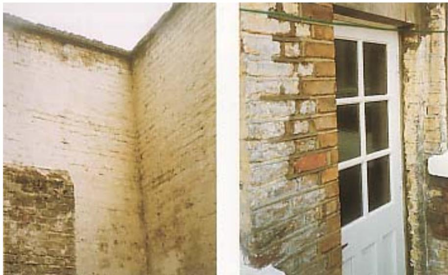
***Gradually the paint deteriorates, blisters and flakes, and the wall may be kept permanently damp. It may facilitate the development of serious infestation, which may need drastic treatment, or even replacement of timber parts of the building or parts of the wall.***
