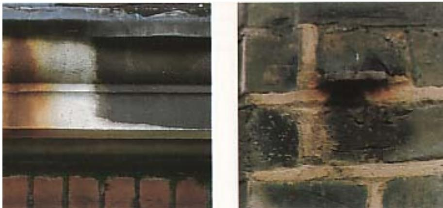
***Examples of metal-corrosion staining on stone and brick.***
