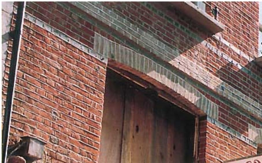
***Dry abrasive cleaning can result in loss of the hard outer surface of brick and/or loss of detail.***
