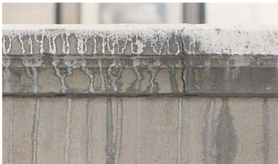
***Acid rain can cause unsightly discolouring of masonry and gradually serious erosion.***
