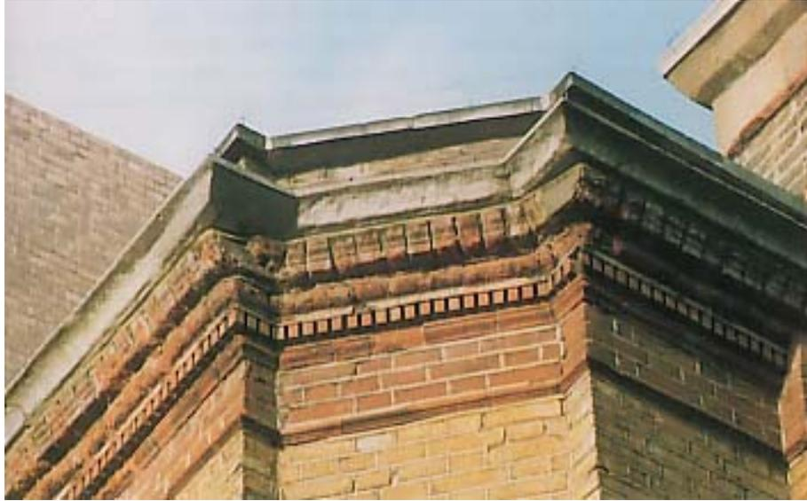
***Eroded brickwork - especially decorative detail - must be properly restored and repointed before cleaning. Pointing must be checked before and after cleaning and, if necessary, repaired.***
