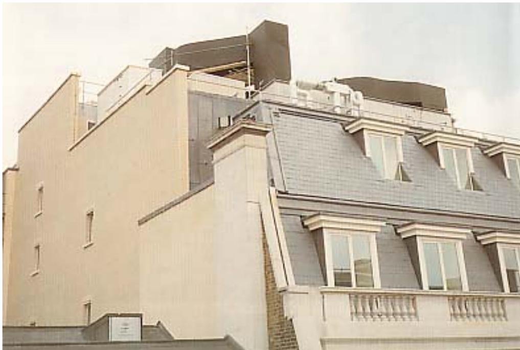
***Air-conditioning plant should always be located out of sight, within the envelope of the roof or screened by an appropriately designed roof-like enclosure. Proposals for new buildings should make adequate provision for plant.***
