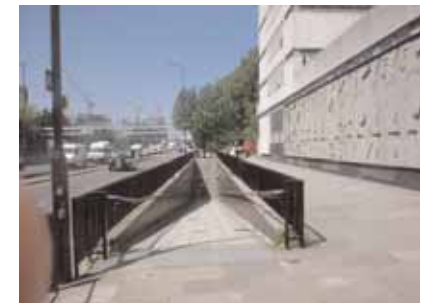
Harrow Road subway
